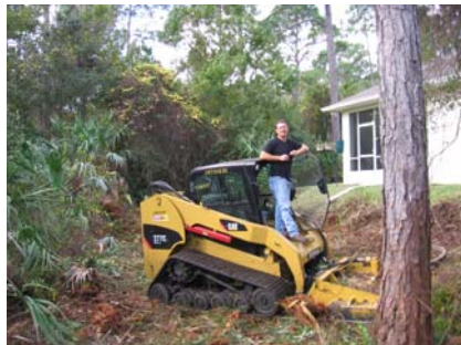
Clearing the fire hazard
