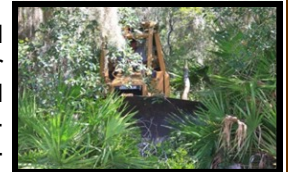
Clearing the roadway
